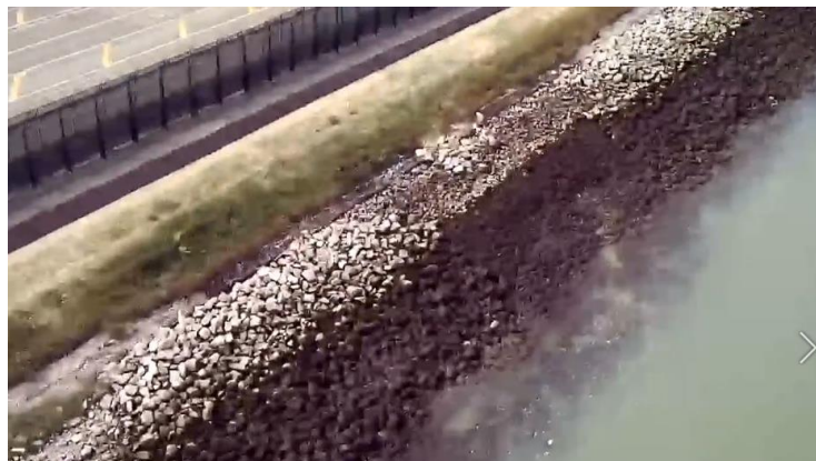
waterways and quays surveillance (outside view)
