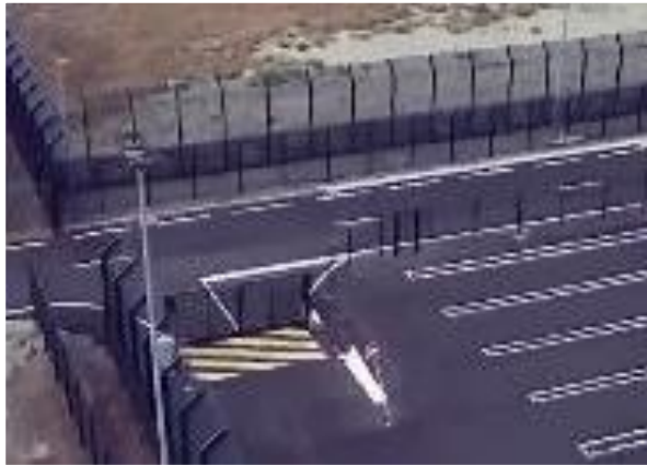
Fence and entrance control
