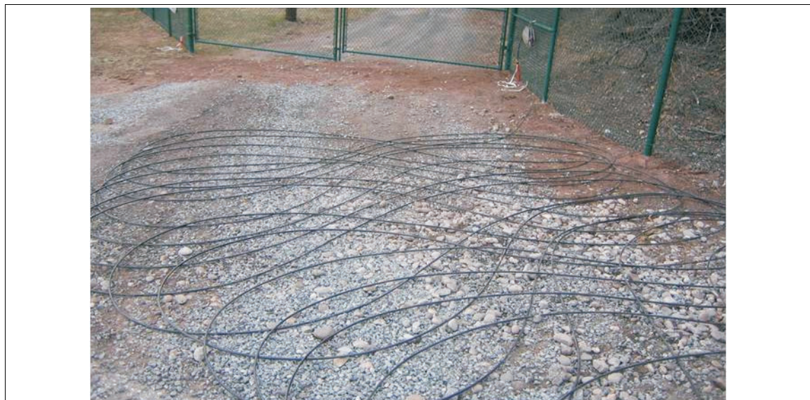
Figure 56 Laying cable in a figure-8 pattern
